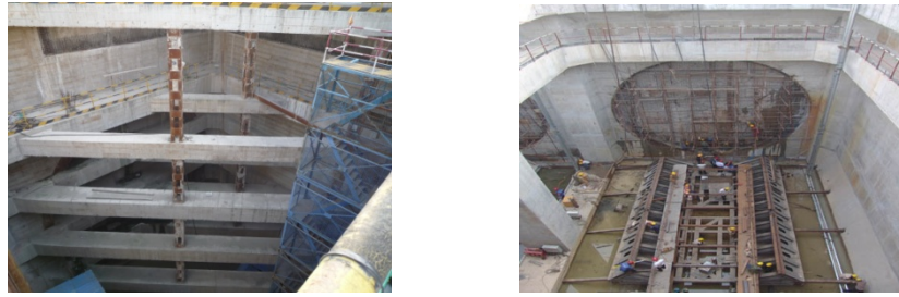
Figure 6.5.2.3-1 Photo of Working Shaft of Shield-driven Tunnel
